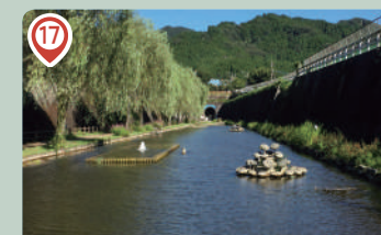
Takamori Yusui Tunnel Park
